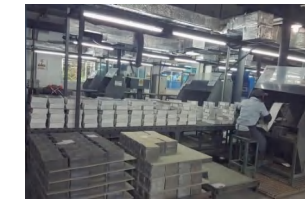
Battery Plates Packing
